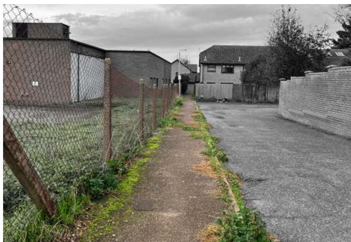
Figure 52: Unwelcoming and therefore underused pedestrian link from residential areas to the High Street
