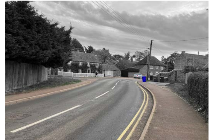
Figure 25 : Fast corner into the High Street with no clear place for pedestrians to cross
