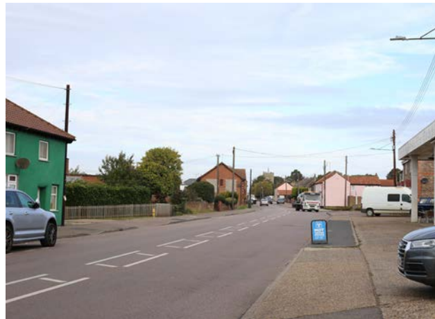
Figure 04: Wide highway encourages speeding traffic along the High Street
