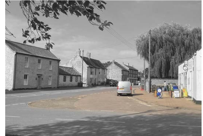
Figure 41 : Large area of low quality hardstanding does not reflect character of Lakenheath
