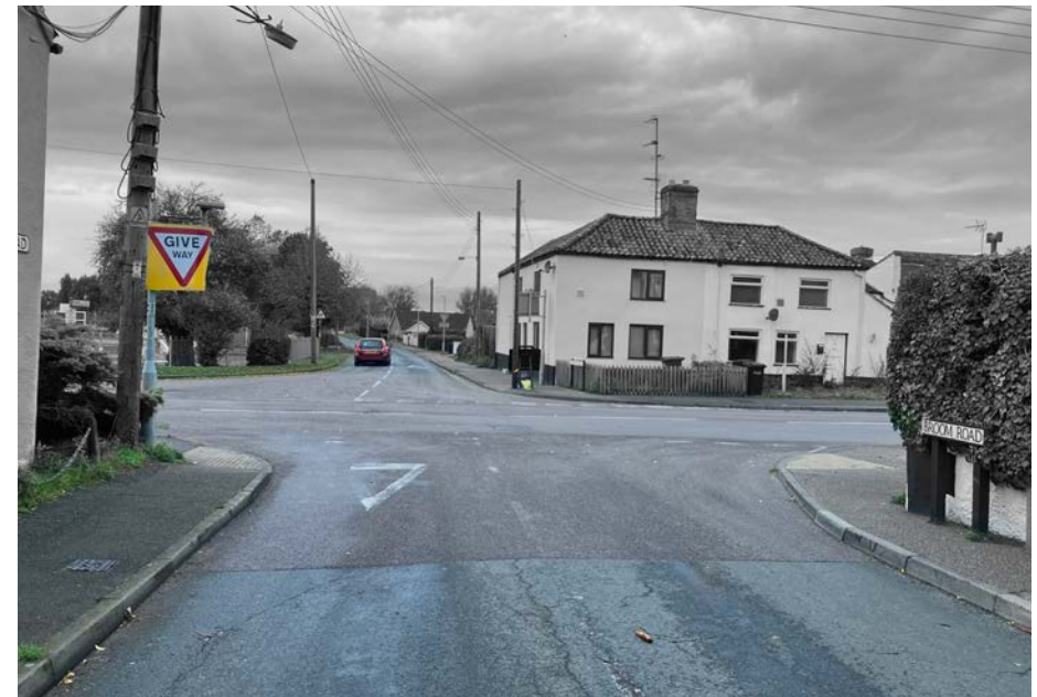
Figure 57: Fast moving junction at intersection of High Street, Eriswell Road, Broom Road and Undley Road, with no designated pedestrian crossing points
