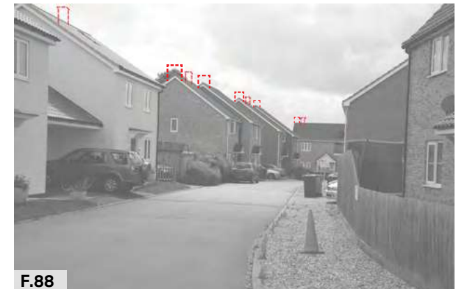
Figure 88: Many recent properties within the Lakenheath Modern Settlement character area don't have chimneys, limiting the interest of the roofline.
