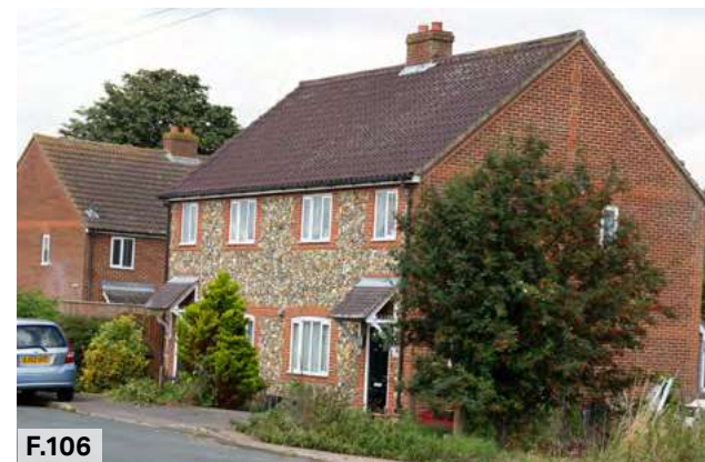
Figure 106: Recent building combines red brick gable ends and window reveals with knapped flint façade.
