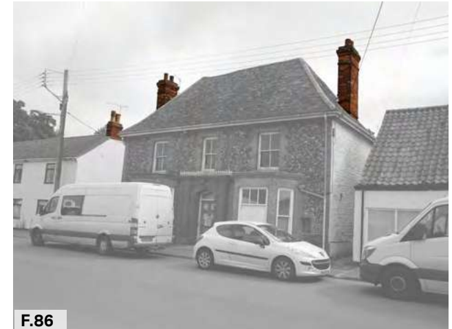
Figure 86: Some landmark properties along the High Street have more prominent ornate chimneys.
