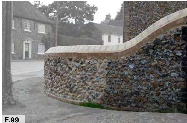
Figure 99: Repaired wall faced with knapped flint and a stone coping in Lakenheath Conservation Area character area.
