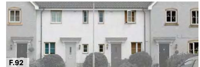
Figure 92: uPVC casement windows in the Lakenheath Modern Settlement character area replicating a traditional sash window form.
