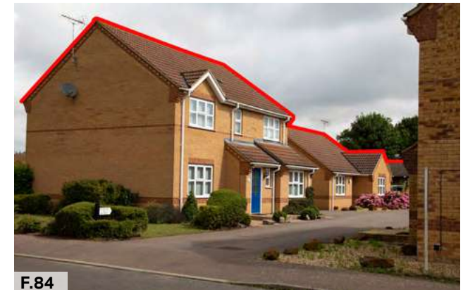
Figure 84: More recent development within the Lakenheath Modern Settlement character area has a wider range of roof types reflecting the form of the buildings.
