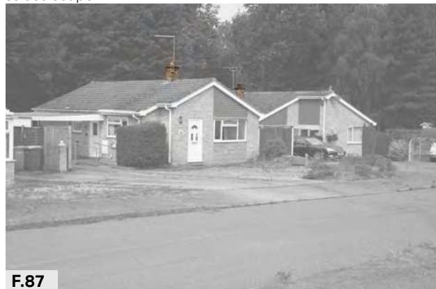
Figure 87: Bungalows within the Lakenheath Modern Settlement character area have simple, functional chimneys.
