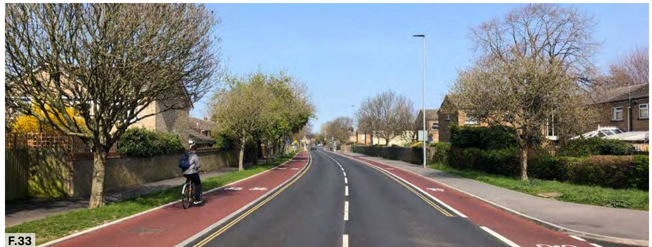
Figure 33: Example of clearly marked out cycle path combined with road within urban context.
