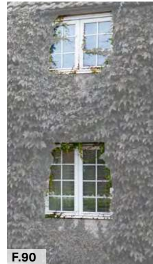
Figure 90: Multi-pane casement windows in the Lakenheath Conservation Area character area.
