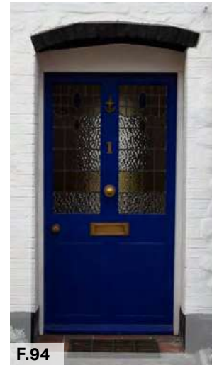
Figure 94: Recessed stain-glass-window panelled door with brick reveal in Lakenheath Conservation Area character area.
