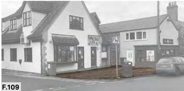
Figure 109: Under-used public / semi-private space outside shops along the High Street.
