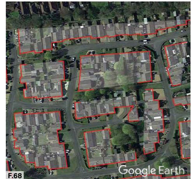
Figure 68: Building set-back vary which provides an interesting street-scape.
