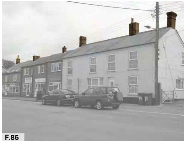
Figure 85: Chimneys are a regular feature along the High Street all with slight differences adding to the sense of variety along the street-scape.
