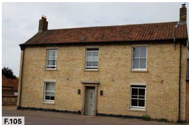
Figure 105: Recently restored yellow brick property on the High Street and Lakenheath Conservation area character area.
