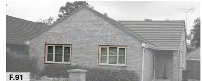
Figure 91: uPVC casement windows in the Lakenheath Modern Settlement character area.
