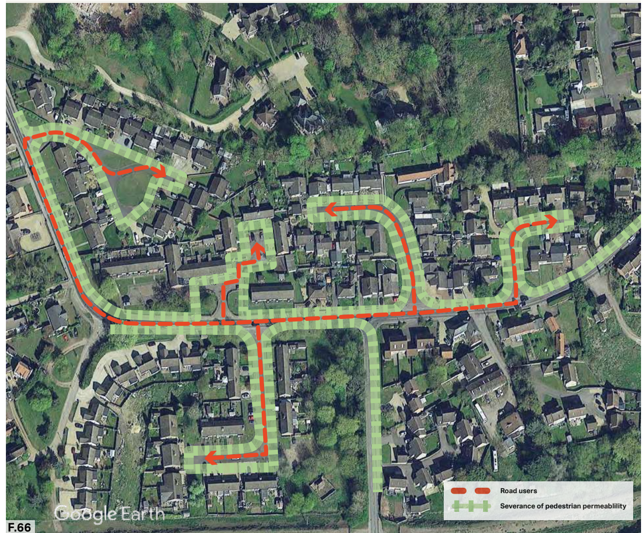
Figure 66: Aerial image of cul-de-sacs accessed from Station Road Lakenheath, illustrating lack of pedestrian permeability.
